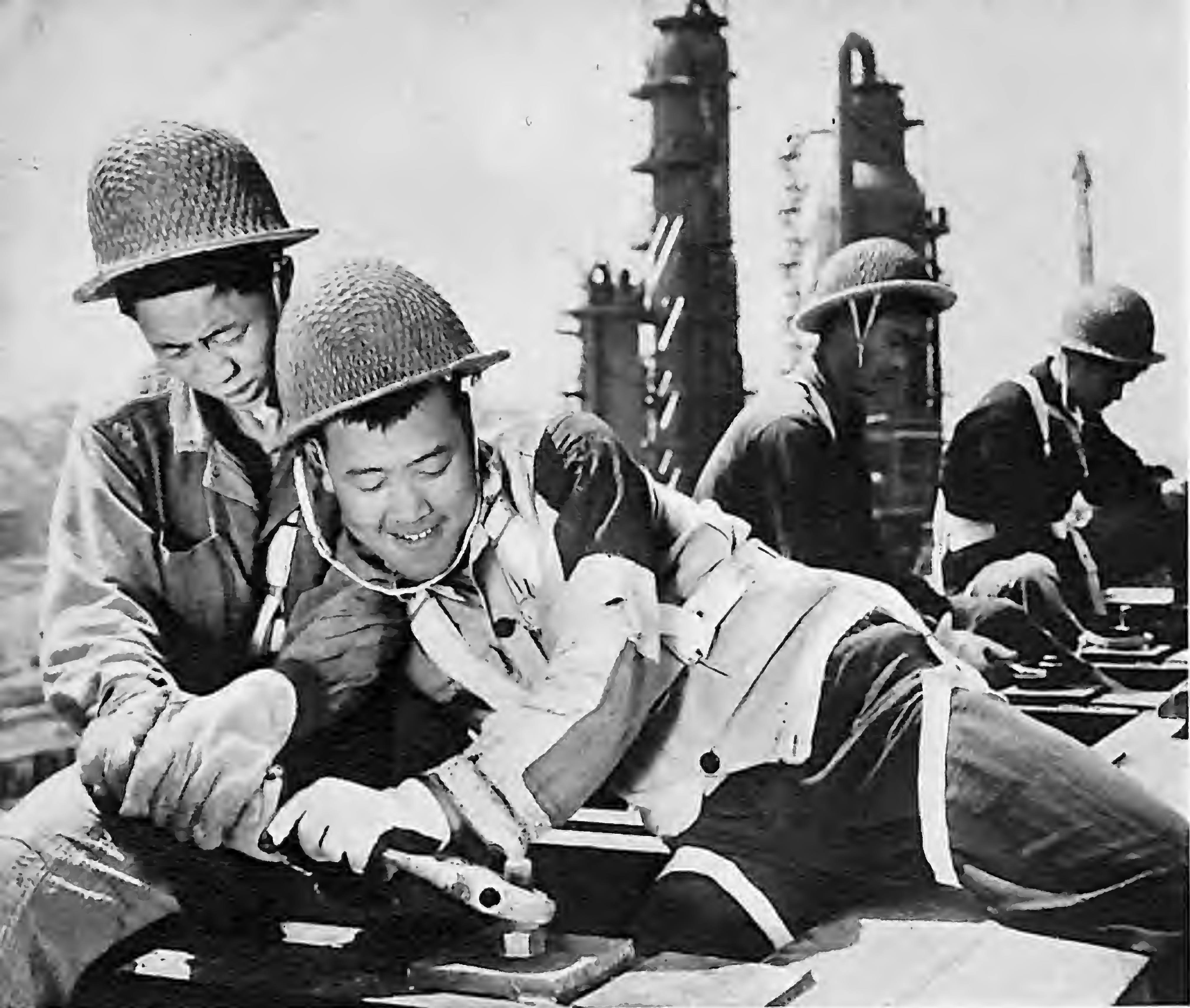
Installing refinery equipment.
